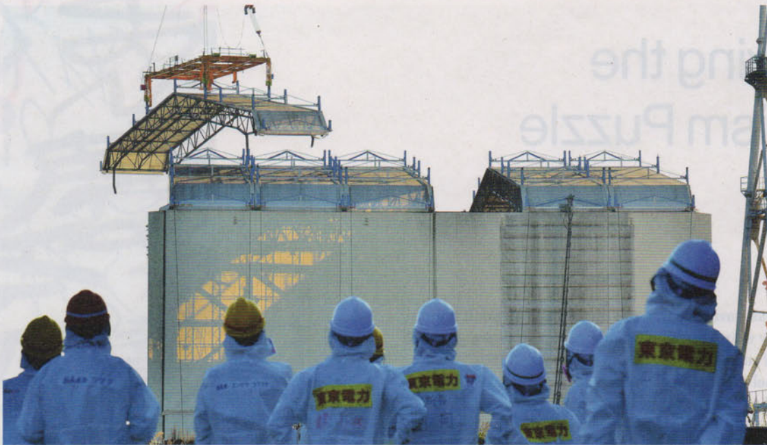
Workers watched in October as a crane lifted a section of a radiation shroud that had been placed over a reactor at Fukushima after the earthquake. Lifting the cover exposed the debris inside the destroyed building for the first time since 2011.
