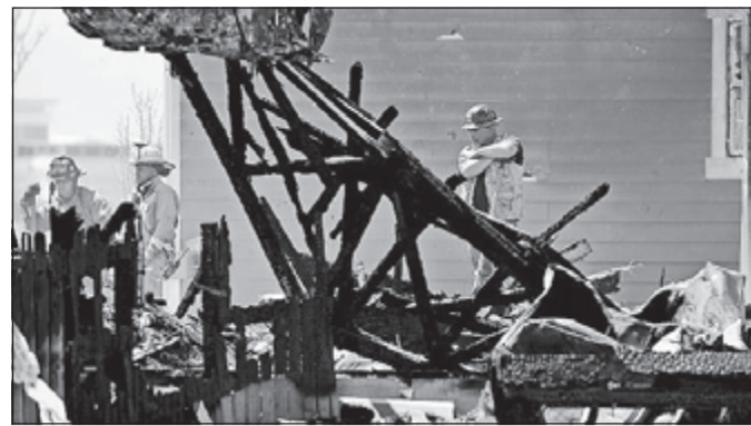
Investigators stand by as debris is removed from a house that was destroyed in a deadly explosion in Firestone, Colo., in April. The home explosion that killed two people was caused by unrefined natural gas that was leaking from a small abandoned pipeline from a nearby well. [DAILY TIMES CALL/MATTHEW JONAS]
