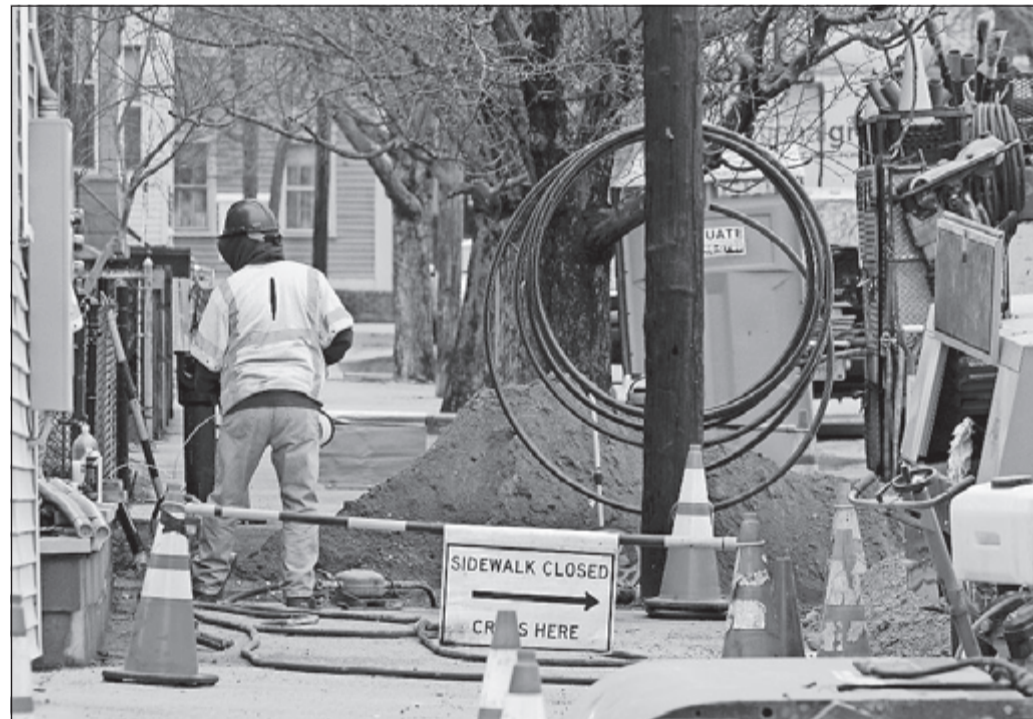
Gas line work being done on Fremont Street in Providence.
