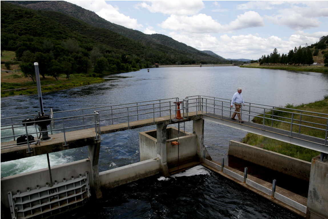
Steven Ritchie, an assistant general manager of San Francisco Public Utilities Commission, walks on a bridge over Moccasin reservoir at the Moccasin Powerhouse in Moccasin, California.
