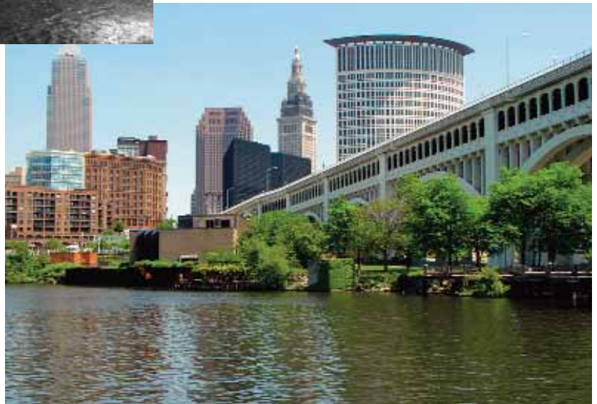
The contemporary Cleveland, Ohio skyline beyond the Cuyahoga River in 2009.
