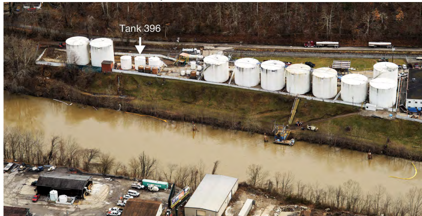
This aerial photograph shows the Freedom Industries tank farm along the Elk River in Charleston, WV. The arrow identifies Tank 396, which leaked the coal-cleaning chemical Crude MCHM into the river on Jan. 9, contaminating the drinking water of 300,000 West Virginians for weeks.
