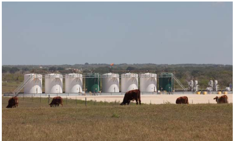
Cattle graze near venting tanks which store produced water (white tanks) and condensate (green tanks) from oil and gas drilling activity nearby. The orange wind sock serves as a protection measure for the poison gas hydrogen sulfide. (Lance Rosenfield/Prime)
