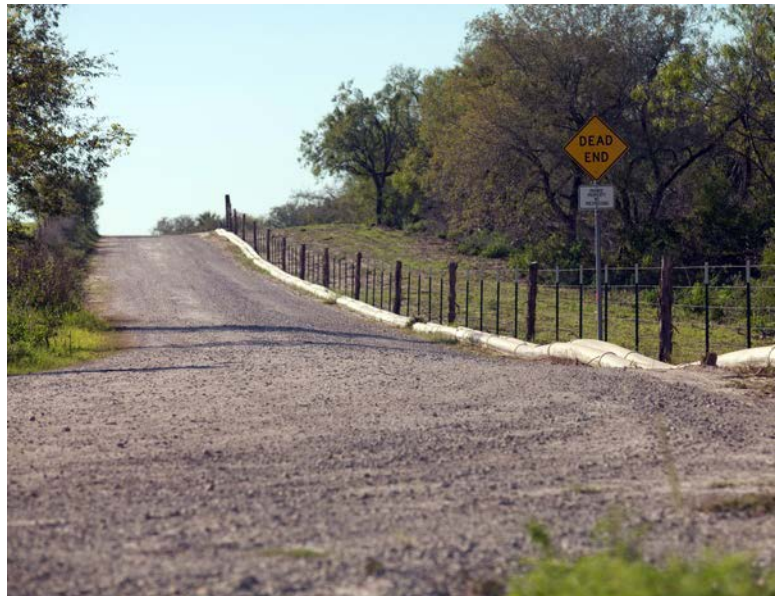
Pipes carrying water for fracking operations line a gravel road in rural Karnes County. (Lance Rosenfield/Prime)
